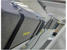
8) After fitting the evaporator box secure the belts and do not overtighten. Make sure there are no gaps around the base of the box.
