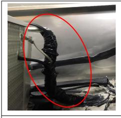
4) Probes and inlet/outlet pipes which connected with Evaporator must cover by PVC insulation tape and make sure all these elements adjust properly.
