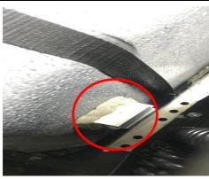
10) Vacuum Breaker must be sealed by putty on Freezer Cabinets, it must be also checked by service technicians!
